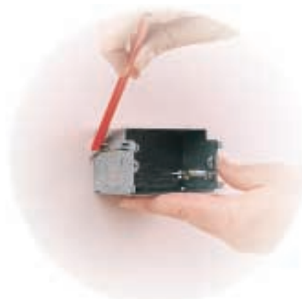
1. Use box to mark cut-out size
